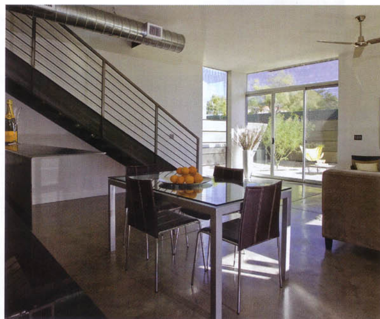
▼ 7" thick post-tension slab provides excellent thermal mass
